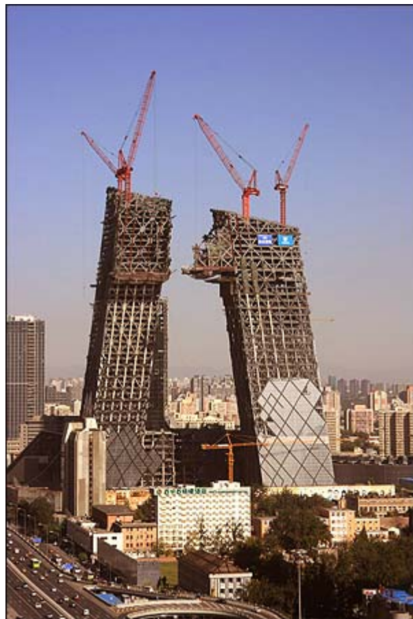
CCTV building under construction.
